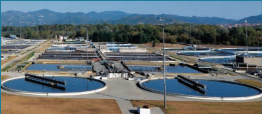
One of the treatment line modules of the Castiglione Torinese wastewater treatment plant.
